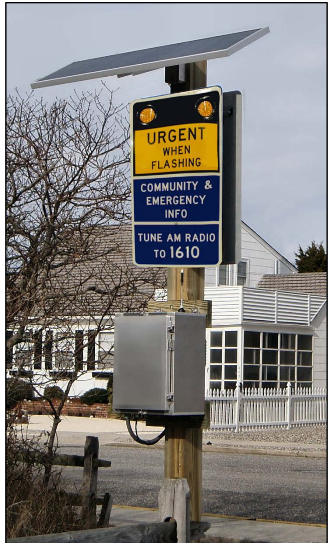
Flash patterns & sign colors comply with the Department of Transportation Federal Highway Administration Manual on Uniform Traffic Control Devices (2004, Regulation 2A.08) . Check with local authorities to coordinate signs in your area.
