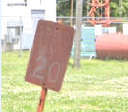
**The damaging effect of salt air on metal – as illustrated by a speed limit sign near the WJOI antenna site.**
